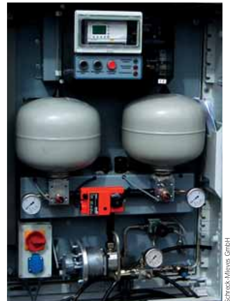
ESA electronic rail lubricating equipment made by Schreck-Mieves.
